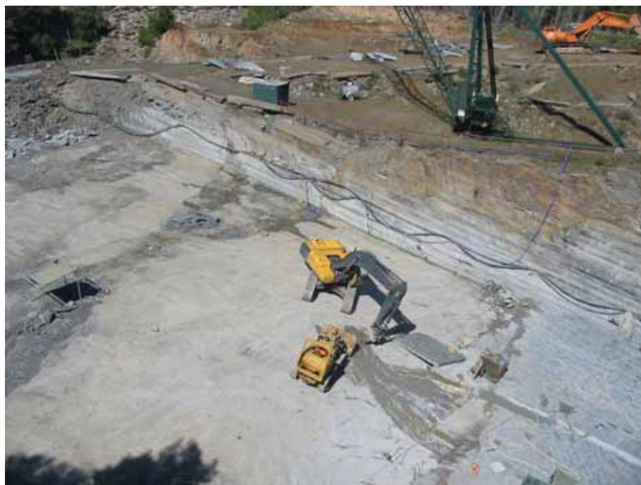
Volvo excavator and front-end loader cleaning the Mintaro quarry floor, which dips gently to the right. A stiff-leg crane on top of the face is about to lift slab to right of excavator. September 2005. (Photo 401879)
