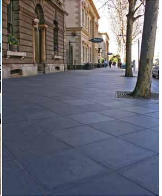
Mintaro Slate used as pavement along King William Street outside the Adelaide Town Hall. (Photo 401878)
